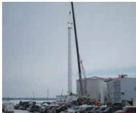
12/18/2008—Setting the Thermal Oxidizer Stack
