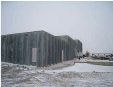
12/15/2008—NE corner of Water Treatment Bldg
