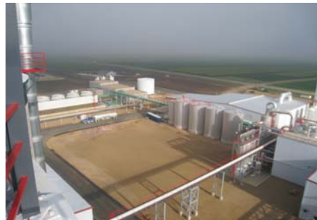
Northwest view from top of silos
