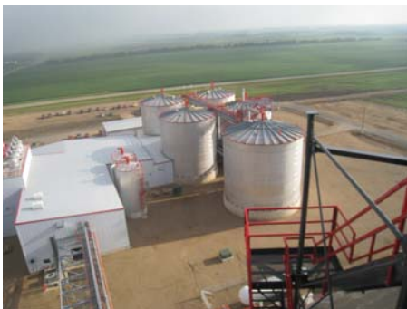
Northeast view from top of silos
