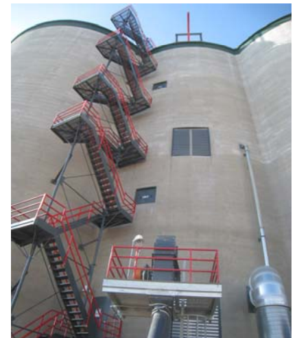
View looking up the silos
