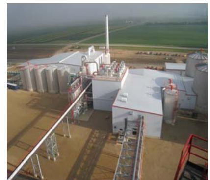
North view from top of silos
