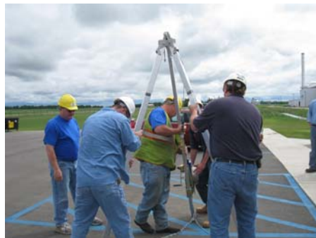
Setting up a safety tripod
