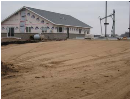
Preparing the ground to do cement work for the scales
