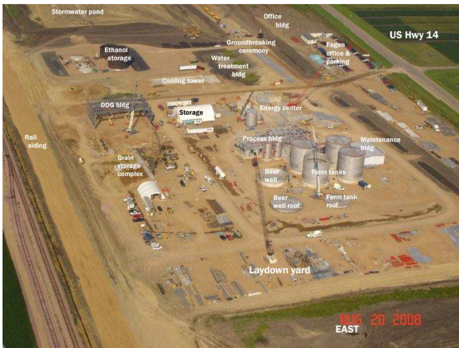
(photo left) Aerial photo taken during the groundbreaking ceremony, August 20, 2008.
