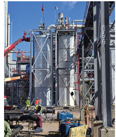
Additional Sieve Bottle Construction - Operational in August 2025
